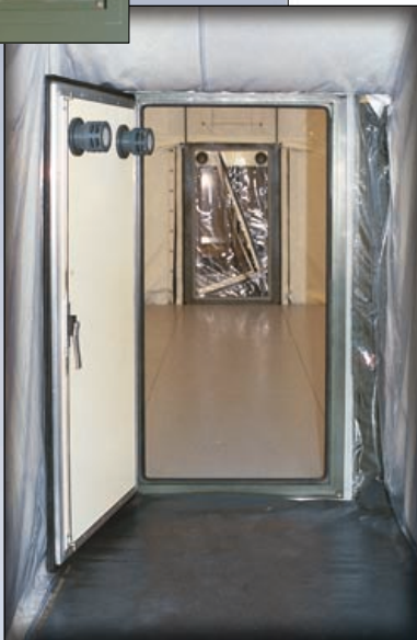
Entrance from the airlock with solid door
